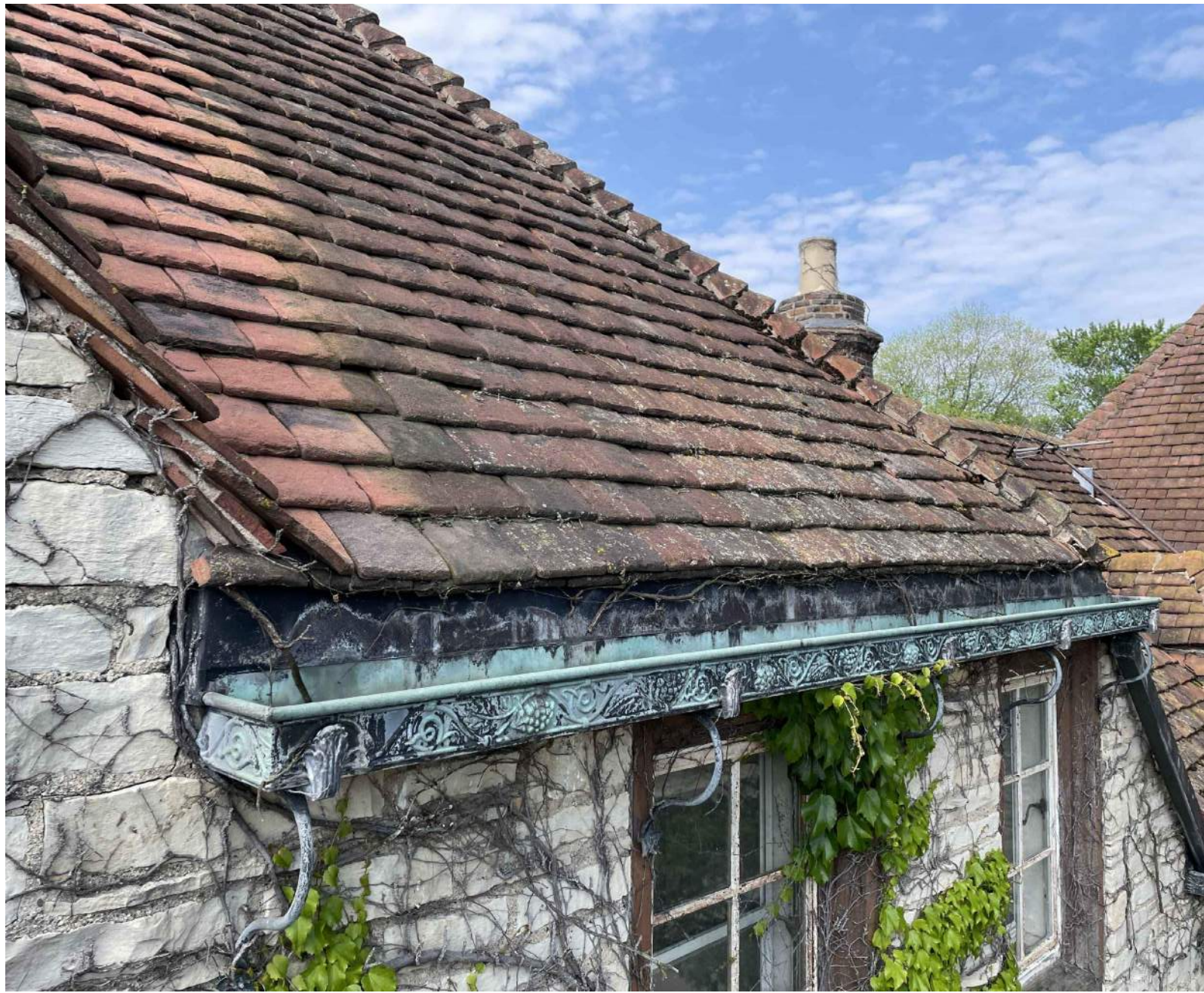
9 TYPICAL COPPER GUTTER SCALE: NONE
